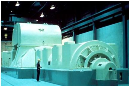
1. Large spinning *generators* produce electricity by constantly moving magnets close to wires.
